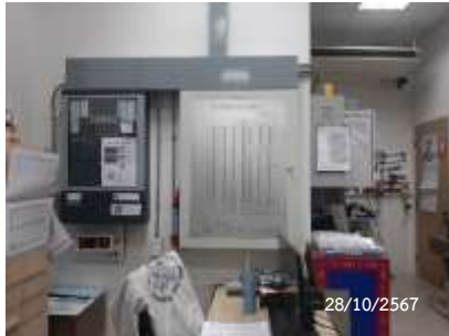
Graphic Annunciator Fire Alarm System
