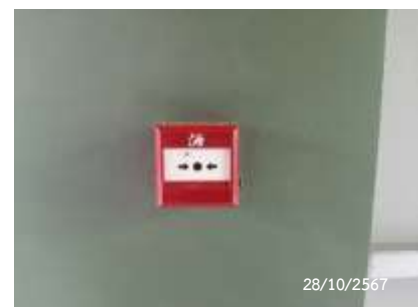
Fire Alarm Manual Station
