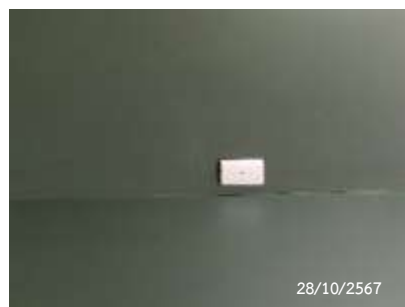
Fire Alarm Indicator Lamp
