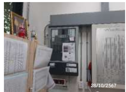
Fire Alarm Control Panel
