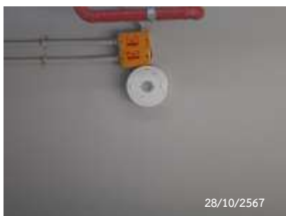
Fire Alarm Horn Strobe
